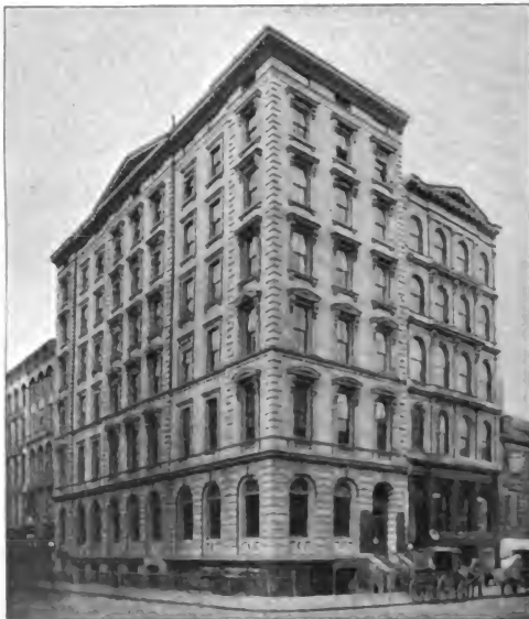
TRADESMEN NATIONAL BANK, BROADWAY, NORTHWEST CORNER OF READE STREET.
